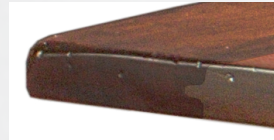
1/2" Breadboard End Detail
