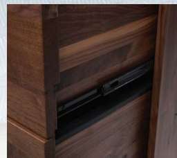
Full Ext Ball Bearing Side Mount Slide
